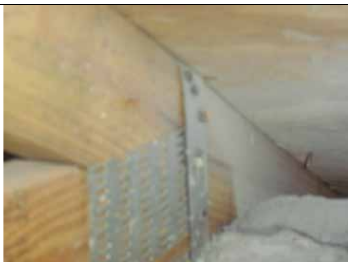
Roof to wall attachment
