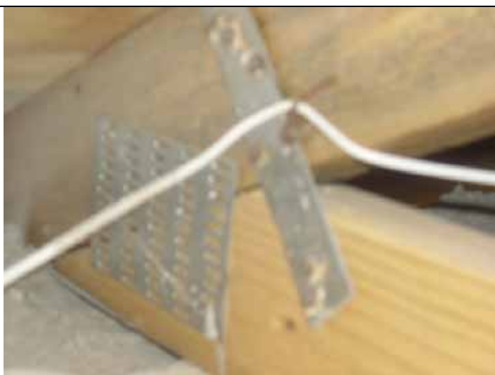
Roof to wall attachment
